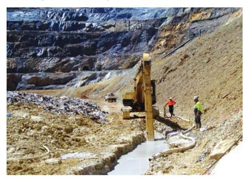
A Cut-off Wall was required to prevent the ingress of very low pH groundwater into the Bioreactor.
