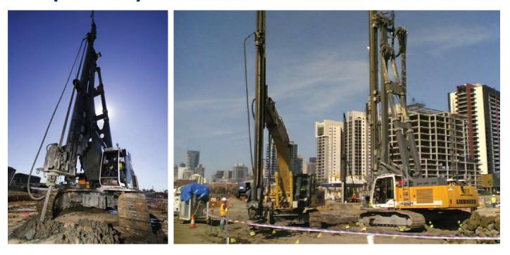
Dry Lime Cement Mixing (LCM) minimised long term creep settlement of the Coode Island Silt subject to increased loads.
