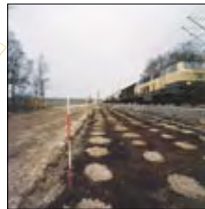
View of the cut off level after Vibro Replacement
