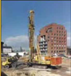
Installation of grouted stone columns with in-situ grouting using cement slurry
