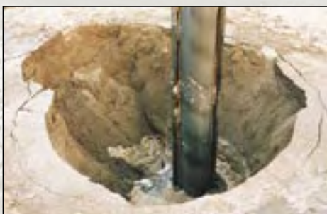
Vibrator in a compaction crater
