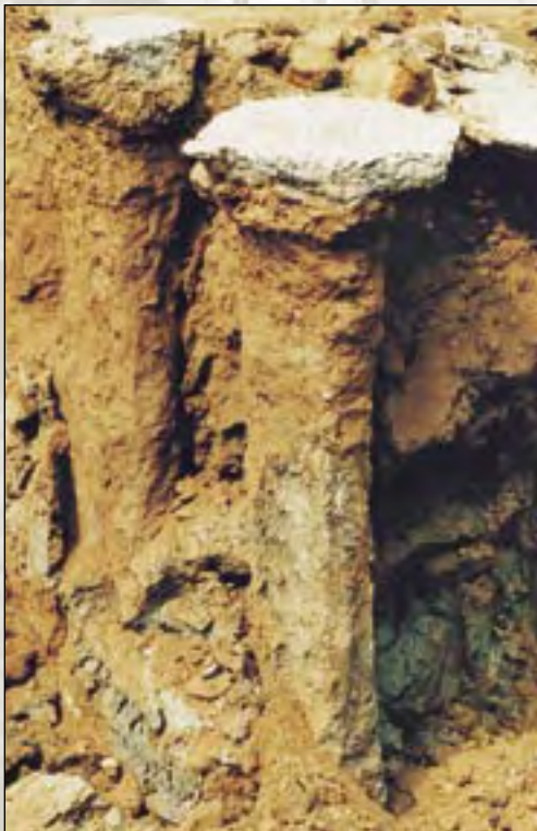
Excavated Vibro Concrete Columns
