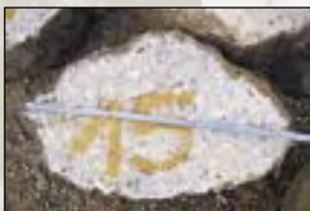
Cross Section of a Vibro Concrete Column
