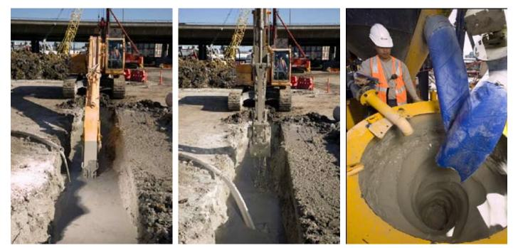
Keller designed a slurry mix to achieve the very low permeability required together with the strain parameters to ensure long term integrity.
