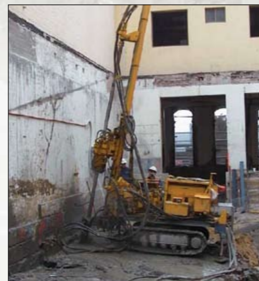
Left: Soilcrete® underpinned Heritage Building, Manly NSW Top: Intimate bond between Soilcrete® and Foundation. Middle: Double or Triple Rods provide separate flows of grout, air and water. Bottom: Jet grout pump.
