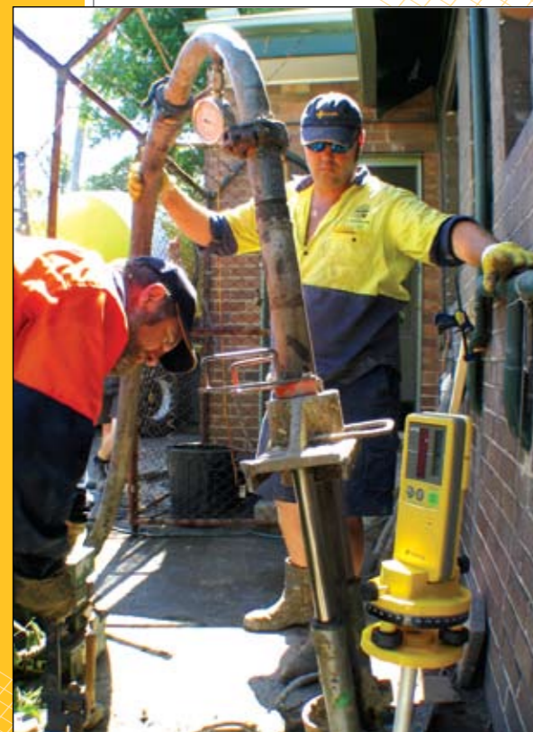
Above: Low mobility compaction grout. Left: Controlled underpinning of shallow foundations.
