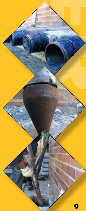
Left: Cone Penetrometer Test results, such as the ones illustrated left for volume cut-off and pressure cut-off, show the degree of improvement achieved by compaction grouting. Right Top: Grout tubes Right Centre: Steel point on driving shoe Right Bottom: Driving grout pipes
