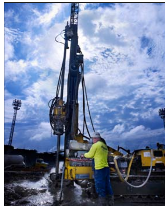
Right: SuperJet Grouting to provide tunnel support at RNA Showgrounds, Brisbane
