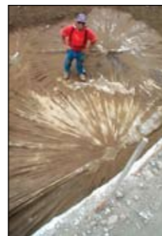
Excavated 5.0m Super Jet Column.
